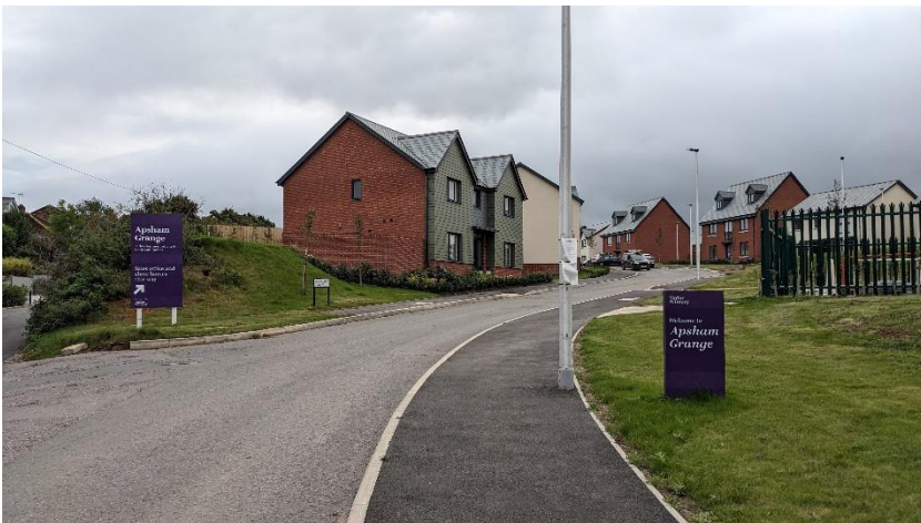
View from Clyst Road, photo shows the Taylor Wimpey housing site
